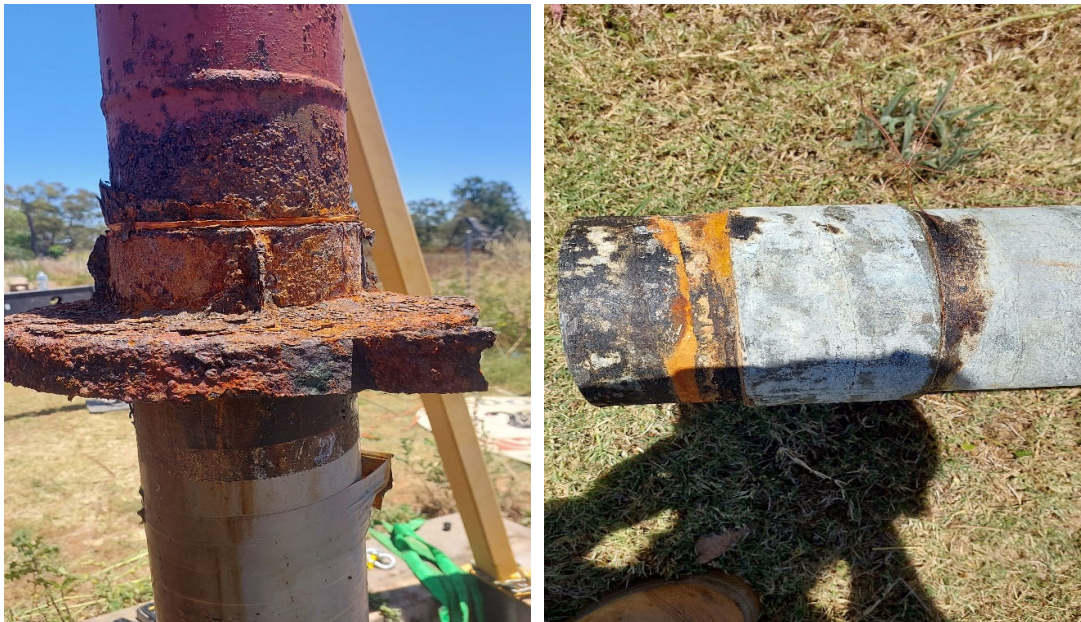
Condition of pumping headworks and column.
