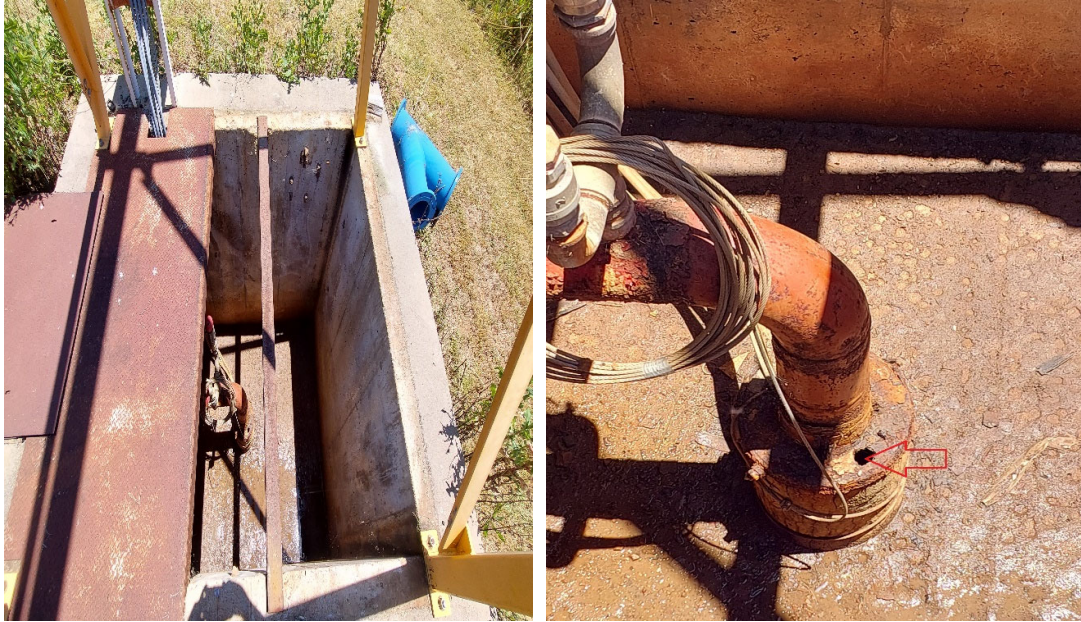
Condition of pumping headworks.
