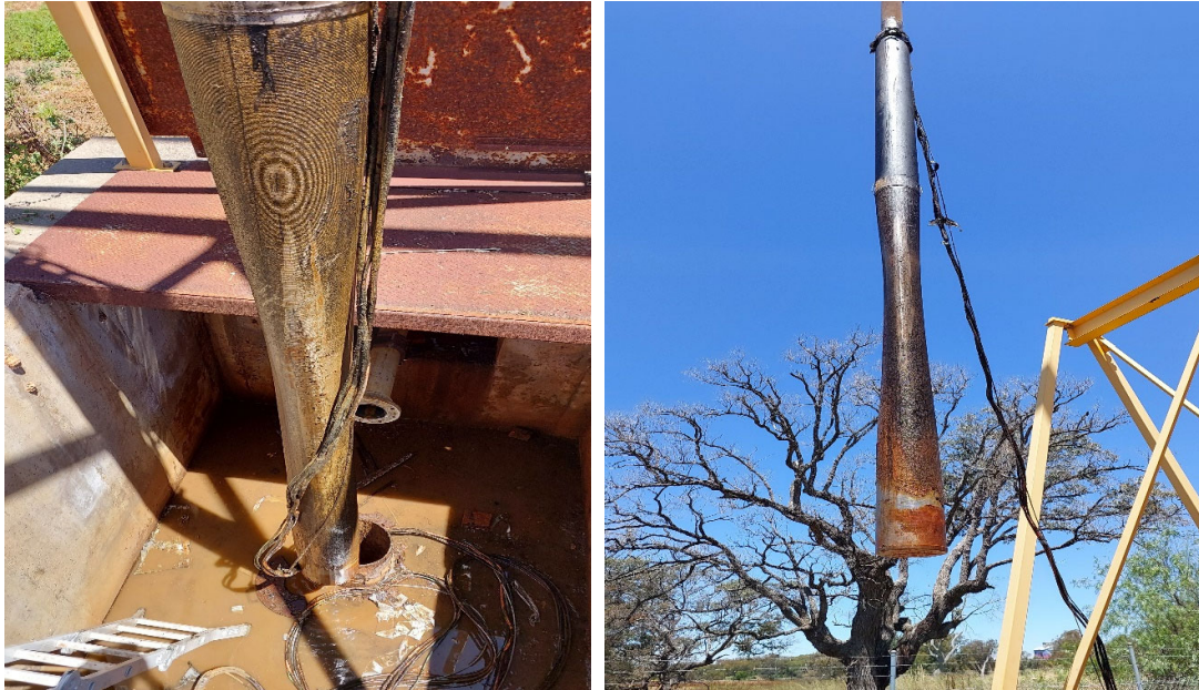
Illustration of stainless-steel screen fitted to pump.
